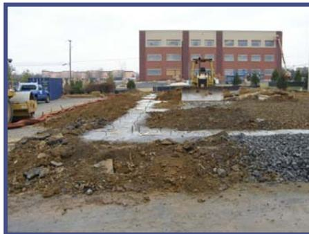
The shop expansion is well underway with the footers in place and the concrete walls scheduled to be set on the 2<sup>nd</sup> week of the New Year.
